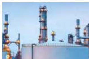
Downstream Oil & Gas (Refining)
